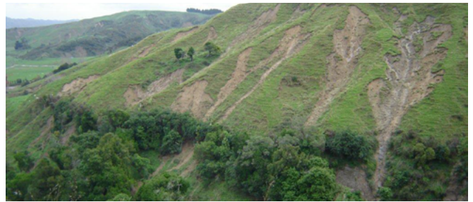
Hill slope erosion following a storm in Wairoa District
