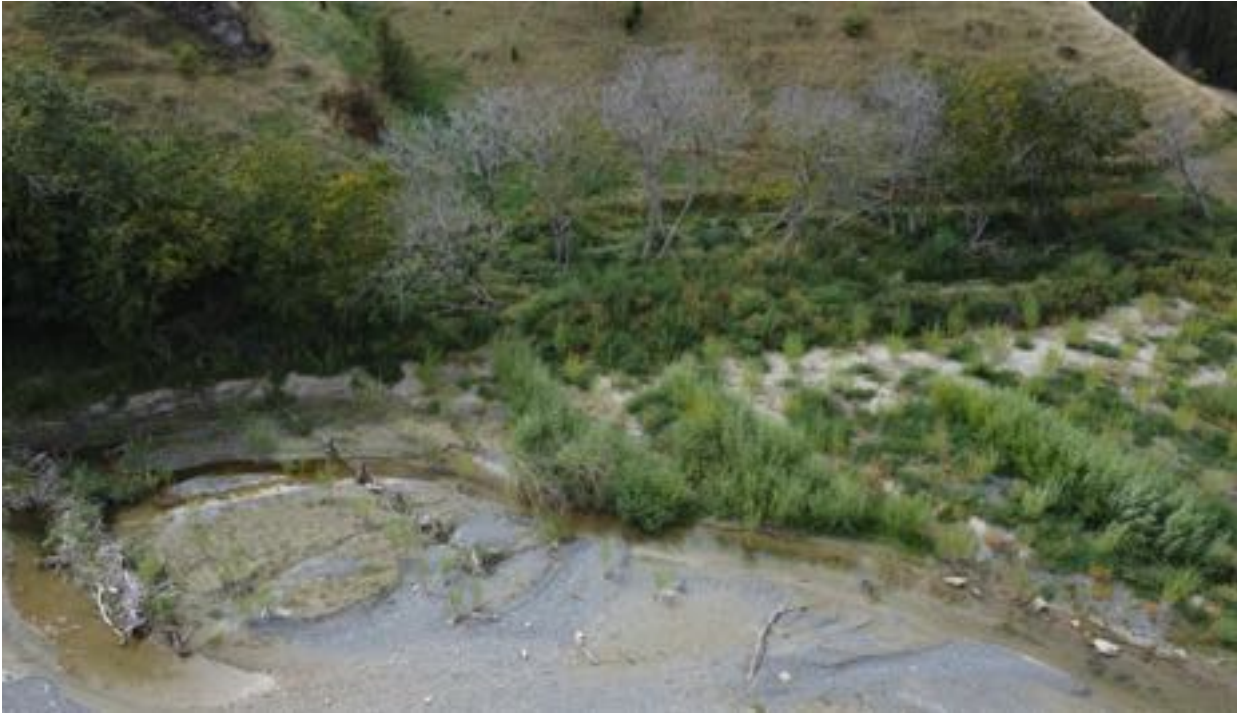
Figure A17. Rope & rail groynes, willow trenching, and pole planting.
