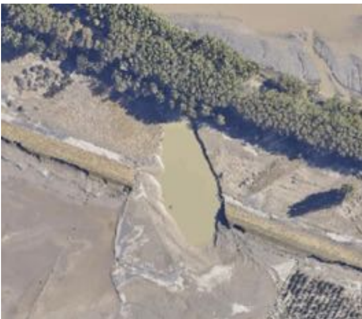
Figure A15. Moteo stopbank breach – berm scour arrested by buffer zone.
