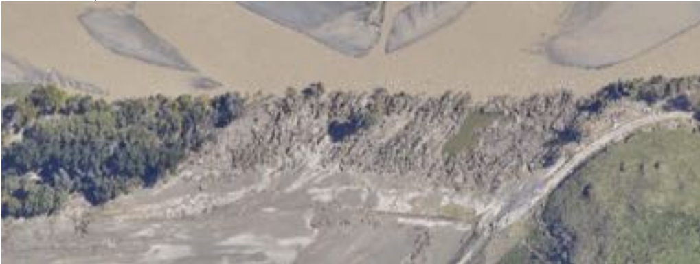
Figure A8. Aerial views of Ebbetts downstream site pre- and post-Cyclone Gabrielle.
