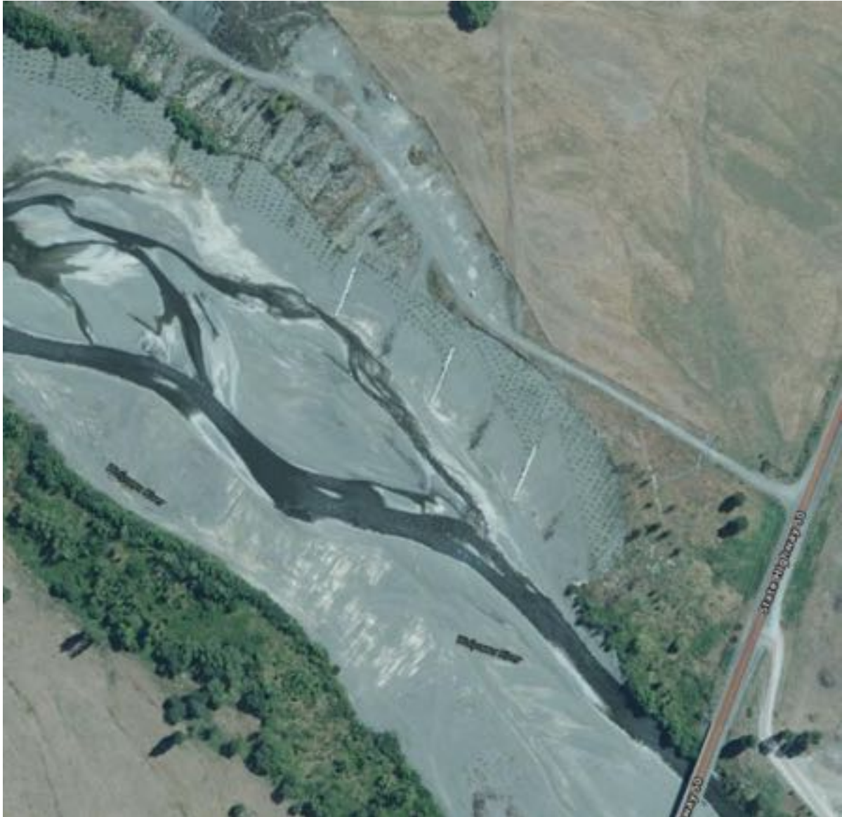
Figure 15. Newly completed Waipawa River training works upstream of SH50 – prior to Cyclone Gabrielle.
