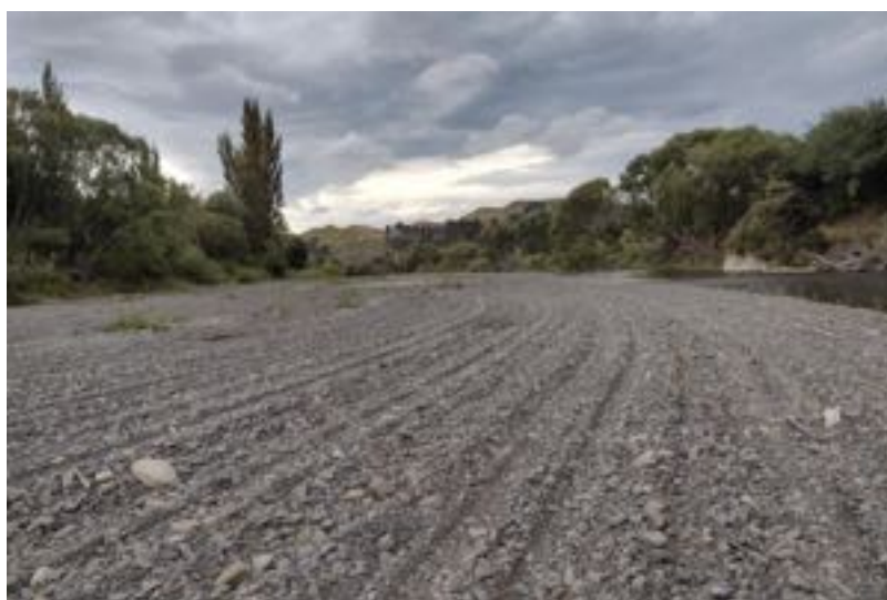
Figure 7. Raking a fairway gravel beach to remove woody and other vegetation, Tūtaekurī River.
