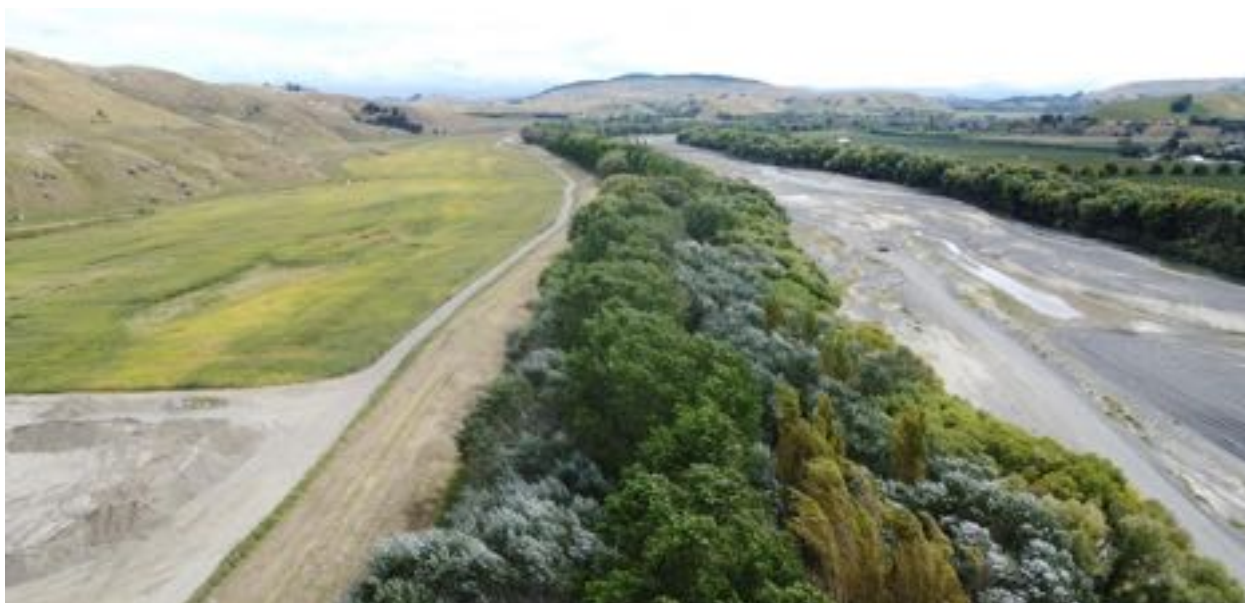
Figure 6. Live edge protection along the Tūtaekurī River. The front edge willows are supported by rows of different poplar cultivars behind.
