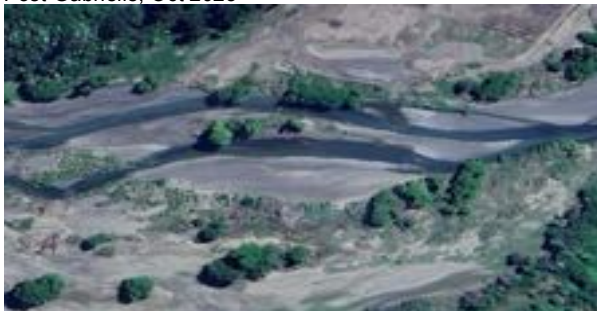
Figure A1. Aerial photos – upstream of Mangaone confluence.
