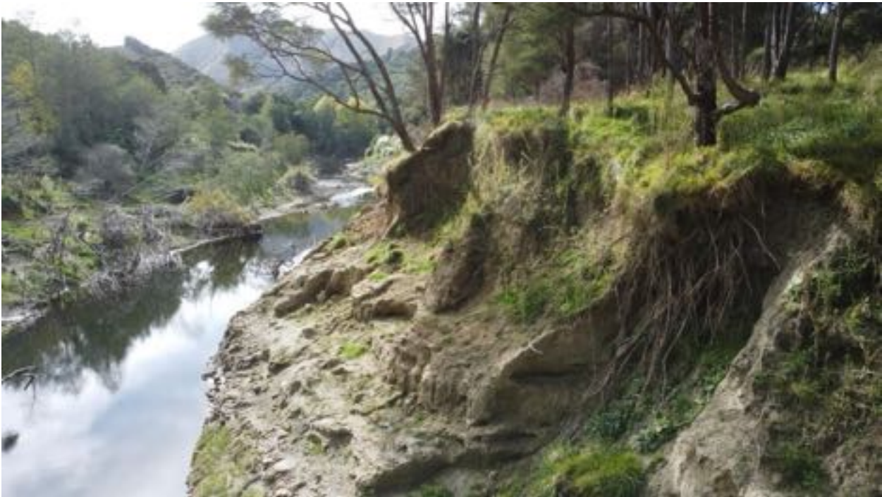
Figure 31. Mānuka roots exposed by bank erosion, Waimatā River. Poplars on opposite side partially destabilised by floodwaters.
