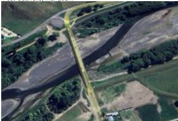
Figure A20. Aerial views of the Redclyffe Bridge.
