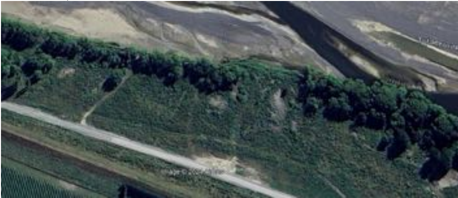
Figure A14. Aerial views of the Moteo site pre- and post-Gabriel.
