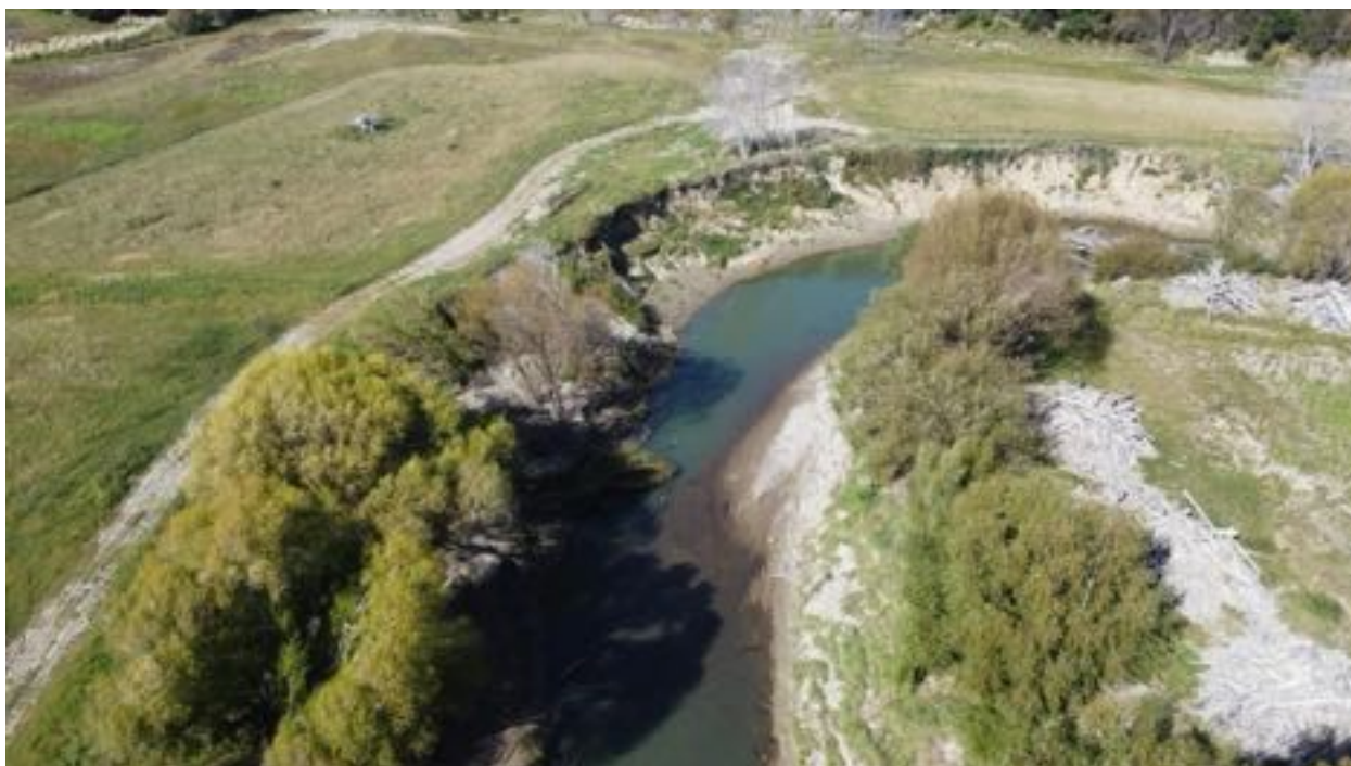
Figure 29. Sparsely treed outer bends showed more toe erosion and slumping.
